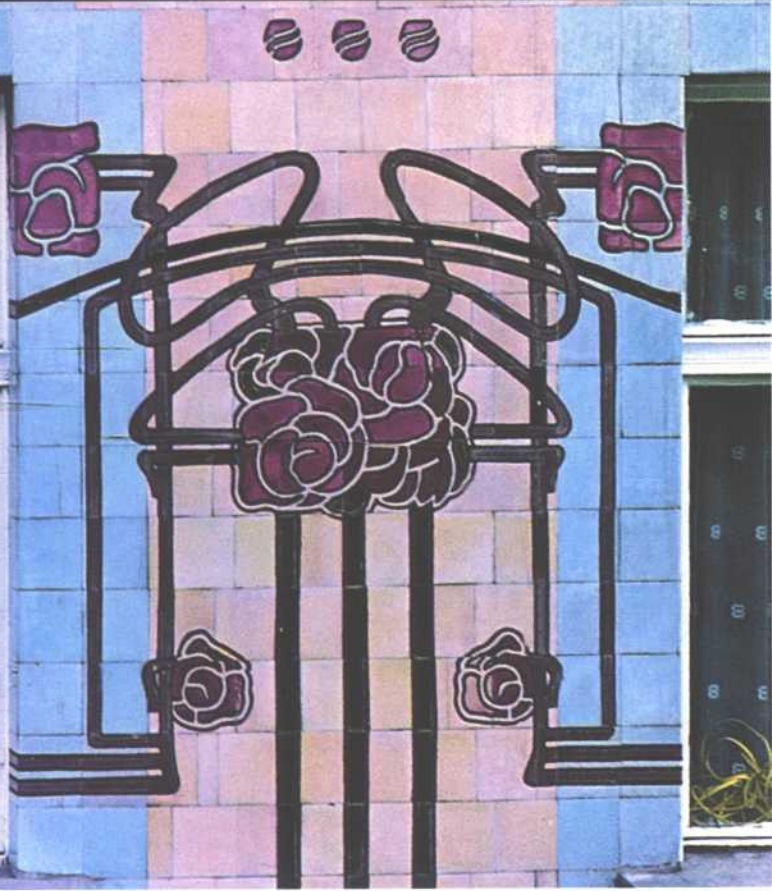
Kalina House Ceramic tiles on façade, V. Bastl, 1903. Zagreb
